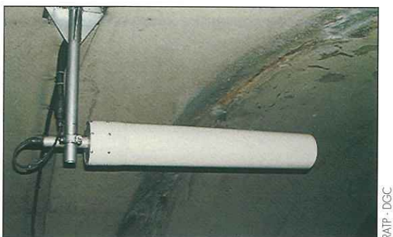
Figure 3. Antenne "yagi".
