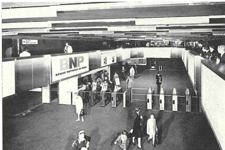
la station HAVRE-CAUMARTIN
